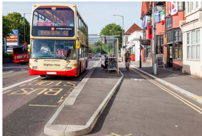
Figure 4.1 Improvements to bus stops along the Lewes Road in Brighton and Hove give passengers a nicer place to wait, but also ensure that traffic along this bus and cycle corridor keeps flowing (Image courtesy of Brighton & Hove City)
