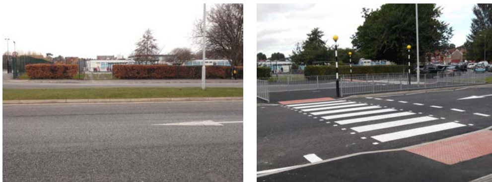
Figure 4.5 Before and after the installation of a double zebra crossing at St John Plessington College in Wirral, identified by students doing a School Route Audit as key to encouraging walking to school (Images courtesy of Living Streets)
